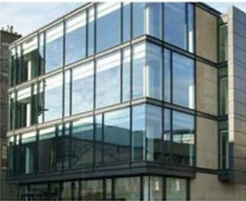
Glazed facade with expressed floor edge
