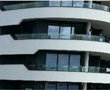
White render balcony parapets
