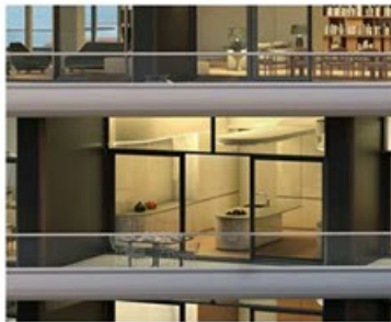
Recessed balcony & glazed balustrade
